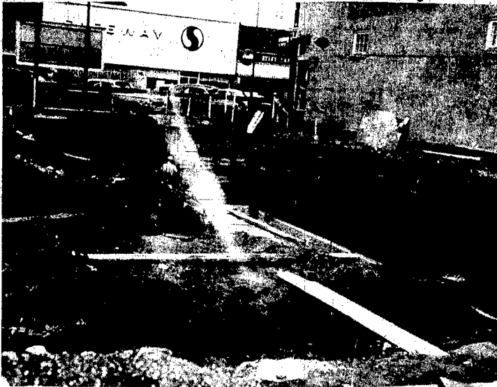
CUSTOMER PARKING AND drive-in banking will be two features incorporated in the new home of the First National bank at Third and Main streets. Workmen are shown here setting forms for the foundation of the 66x39 building. An additional service will be two night depositories, with an envelope drop for individuals and a bag drop for merchants. Completion is expected in November.
