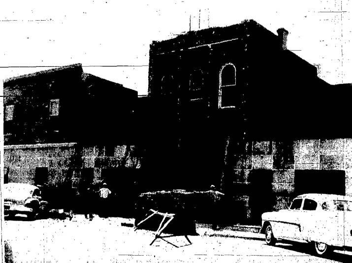
MORE SPACE AND drive-in banking services will be added to the State National bank when workmen complete the project shown here. The expansion is being added to the west end of the present building and will take in the space formerly occupied by the Economy market and Bressler Feed and T.V. Drive-in banking will be provided in the area under the two-story portion of the addition.
